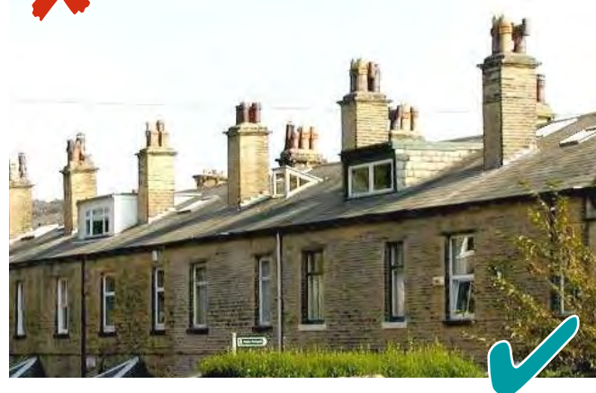
Top: Only two of the nine houses in this terrace retain all their details giving a disjointed skyline. Above: The retention of full height chimneys and pots gives this terrace a uniform appearance.
